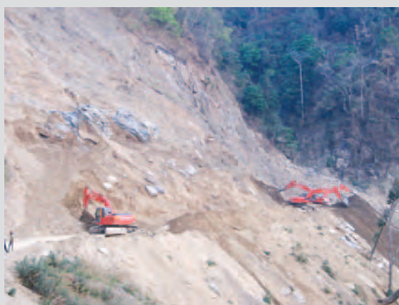
The highway construction passes through steep terrain
