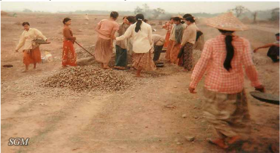
Villagers forced to assist in road construction in Arakan State
