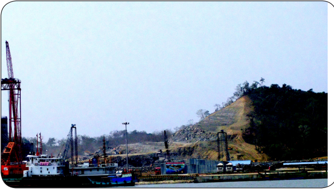
Construction on seaport in Kyauk Phyu
