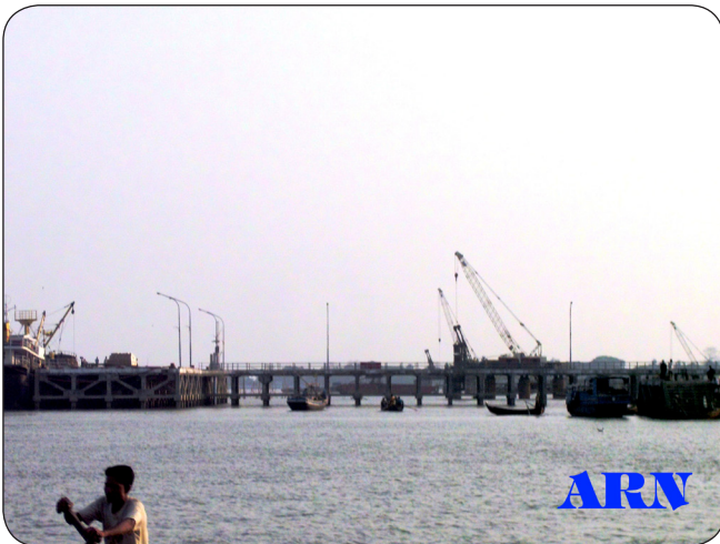
View of Kaladan Multi Modal Transit Project construction in Sittwe
